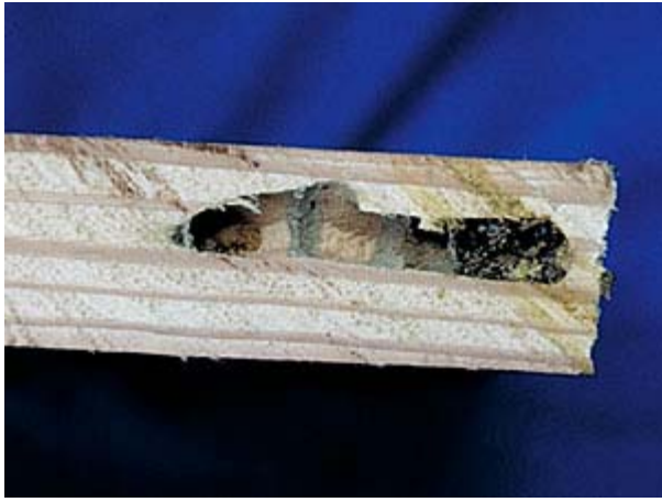
Carpenter Bee Tunnel
